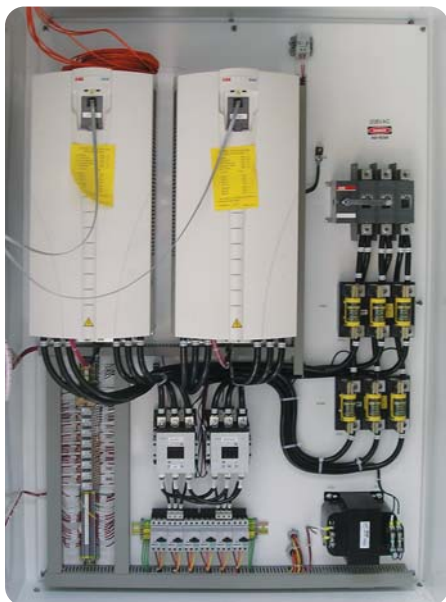
The unit control panel includes redundant variable-frequency drives for the fan motors. This ensures heightened system reliability. The panel also includes circuit protection equipment and system interfaces with building automation systems using standard protocols.
