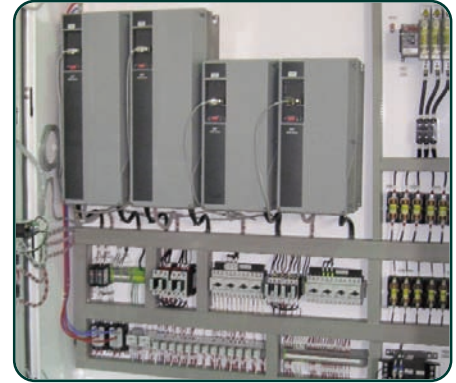
Factory wired control panels from HUNTAIR with redundant VFD drives for supply and return fans.
