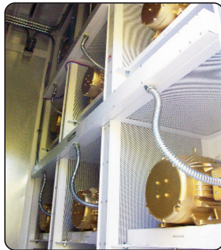
Nine-fan array of one of the 34,000 CFM HUNTAIR air handlers providing reliable airflow through redundant FANWALL cells.
