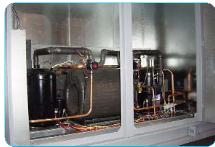
Ground-coupled heat pump comes factory packaged inside ventilator minimizing start-up time.
