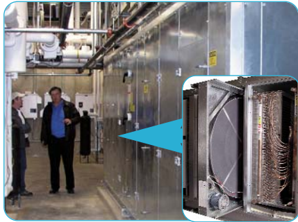
Dedicated outdoor air ventilator uses an AHRI Certified™ total-energy wheel to recover energy between the exhaust and outdoor airstreams.
