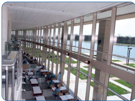
Sherman Hospital takes full advantage of natural lighting and features numerous advanced design elements for energy efficiency as well as optimized work flow.
